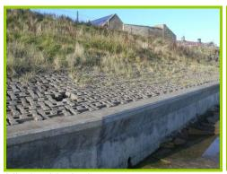
Missing block along concrete revetment at south end of Cresswell.
