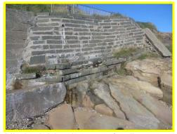
Missing bricks along toe of wall supporting access ramp.
