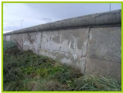
Minor cracks to in the seawall to the south of the access ramp.
