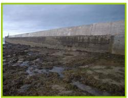
Repairs to crest of North Sunderland Harbour breakwater in good condition.
