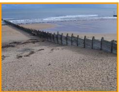
Gaps between groyne planks and low Arson damage beach levels in the lower/ middle beach. of the seawall.
