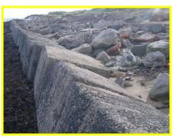
Some displacement and gaps in concrete block 'wall'.
