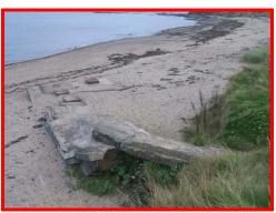
Dilapidated outfall requiring removal or repair.
