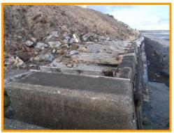
Erosion of slopes behind timber breastwork and exposure of tie-backs.
