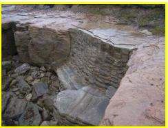
Abrasion and undermining of toe of localised masonry/ concrete walls.
