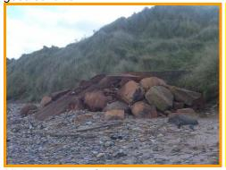
Highly rusted outfall in need or repair or removal.
