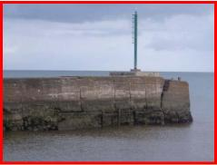
Large crack and rotation of tip of North Pier.
