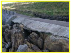
Gabion baskets at the bottom of the access ramp have split.
