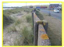
Some rotation of concrete post and plank wall at back of dunes.
