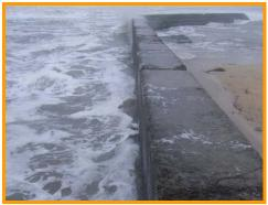
Abrasion and cracking to Green's Haven Damage to Crest of Green's Haven Breakwater.
