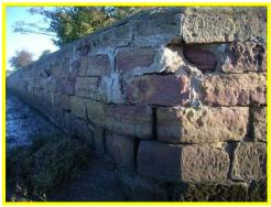
Cracking and missing pointing at the corner of the wall along the footpath.
