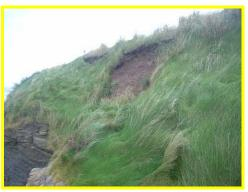
Erosion of upper earth cliff at east end of seawall due to overtopping.
