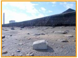
Very active erosion of tipped colliery spoil releasing waste onto the foreshore.
