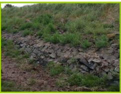
Some gaps in asphalt and stone revetment to flood embankment.
