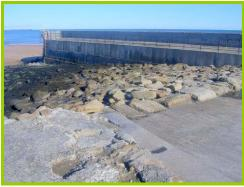
Grouted stone revetment in lee of pier in Undermining of toe at seaward end of good condition.
