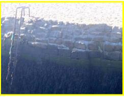
Repairs undertaken to gaps between blocks in masonry wall.
