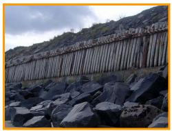
Broken and missing timber boards and rotten wailing beam to breastwork
