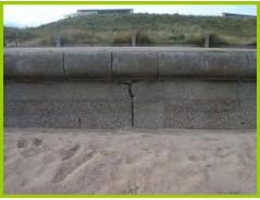
High beach levels, minor cracks and gaps at construction joints.
