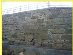
Gaps and some larger holes between blocks in masonry seawall.
