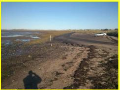
Localised erosion damage to road at Chare Ends
