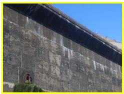
Loss of mortar beneath the coping along Full height gaps in the brickwork in the most of the wall.
