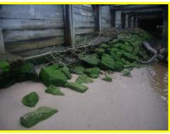
Displacement of stones and unravelling of masonry toe at Spittal Quay.
