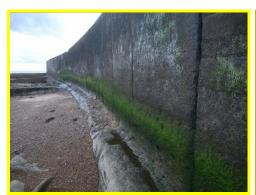
Abrasion of toe, vertical cracks and gaps Significant horizontal cracking, spalling in joints at the East Pier seawall.
