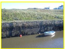
Missing mortar and gaps between blocks along eastern harbour quaywall.
