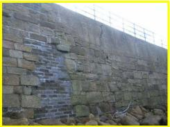
Cracks in upper section of masonry seawall on Rocky Island.
