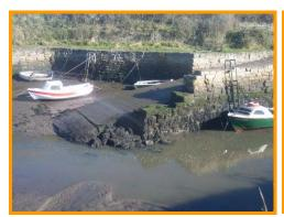
Some missing blocks and rotation of outer wall of slipway.
