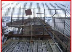
Gate and missing section of timber walkway preventing access to seaward 2/3<sup>rds</sup> of structure.
