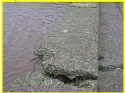
Exposed reinforcement in cope.
