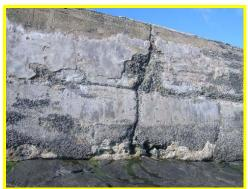
Full height crack and voids at the toe on Cracks to the surfacing on the south the south harbour arm.
