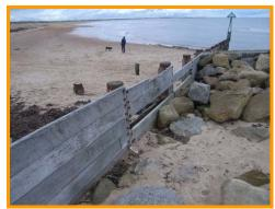
Missing planks and damage to timber groyne at mouth of Seaton Burn.
