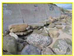
Low beach levels causing undermining at toe of seawall north of access ramp.
