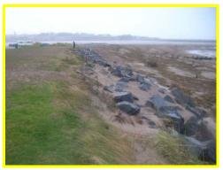
High beach levels burying revetment and windblown sand on embankment.
