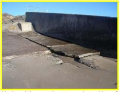
Undermining, settlement and cracking of to concrete apron adjacent to ramp.
