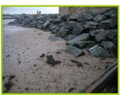
Accretion of sand burying toe of revetment.
