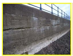
Horizontal cracks along South Pier highly abraded.
