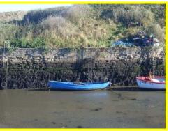
Settlement, abrasion and missing mortar in masonry quaywall.
