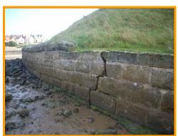
Full height vertical cracks in joints and blocks in masonry wall at Church Hill.
