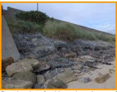
Deterioration of gabions along the toe of the dunes.
