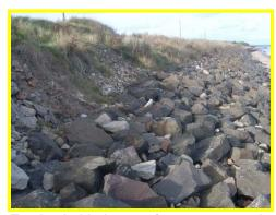
Erosion behind crest of revetment south of Low Hauxley.
