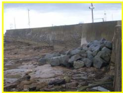
Abrasion and scour holes along seaward face of Main Pier and flattening of rock armour profile.
