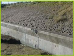
Minor abrasion to low concrete wall at south end of Cresswell.
