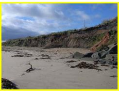
Erosion of earth cliffs and outflanking of revetment at south end.
