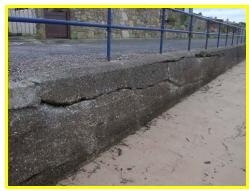
Horizontal cracks along the cope of the seawall at Bay View Road.
