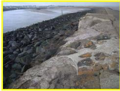
Some movement of smaller armour stones and gaps in pitched stonework on south face of North Pier.
