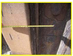
Corrosion of steel piles resulting in noticeable loss of thickness.
