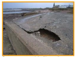
Damage to crest slab of low wall at Newbiggin Point.
