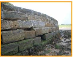
Cracks and displaced blocks causing significant loss of retained material.
