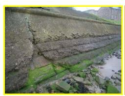
Abrasion of concrete casing exposing masonry blocks on Pier Road seawall.
