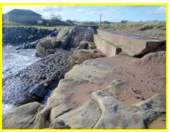
Slight undermining and outflanking of old concrete outfall at Spital Point.
