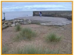
Undermining of concrete deck at harbour arm.
