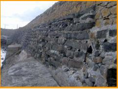
Serious deterioration of the seaward side of the masonry seawall.
