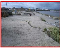
Failed section of Broom Hill quay with significant settlement/ cracking of deck.
