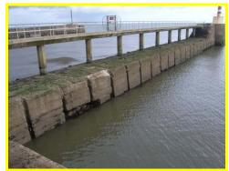
Significant abrasion to the base of the South Pier Head.
