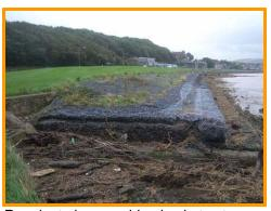
Repairs to lower gabion baskets at south end of structure.
