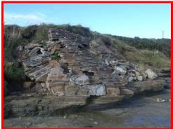
Obsolete masonry revetment south of Snab Point continues to break up.
