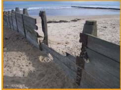
Arson damage to the first groyne south of the seawall
