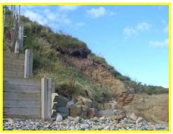
Some erosion along northern edge of retaining wall could lead to outflanking.
