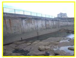
Localised cracks, rust staining and spalling along the wave wall.
