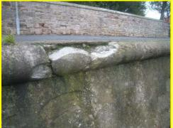
General cracking and spalling to the cope.
