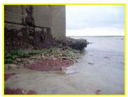
Undercutting of the toe apron at the head of Beadnell Harbour breakwater.
