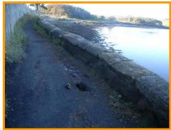
Void in footpath, possible caused by loss of fill through gaps in masonry wall.
