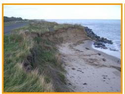
Outflanking of the revetment south of the Hadston Scaurs slipway.
