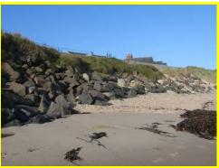
Some erosion behind crest of revetment north of Cresswell.
