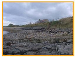
Burst baskets along the toe of the gabion revetment at Ladies Hole.
