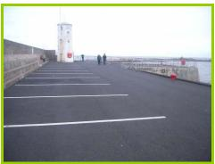
No settlement or cracking evident in new surfacing to Main Pier.
