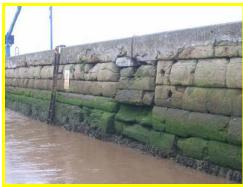
Abrasion and cracking of masonry blocks on west face of Spittal Pier.
