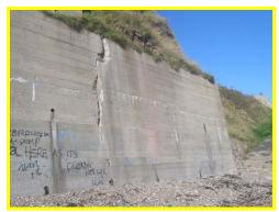
Notable vertical crack in high seawall at centre of the bay.
