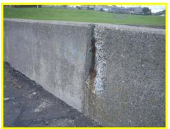
Spalling and rust staining to the setback wall.
