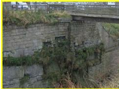
Gaps and missing blocks in the masonry Partially collapsed sections and further wall along the man-made channel.
