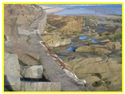
Exposed reinforcement along crest of wall at Cresswell.
