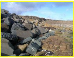
Erosion and outflanking at the north end and placement of smaller armour rocks.
