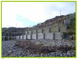
Timber retaining wall improved in 2010 to prevent slips in upper slopes.
