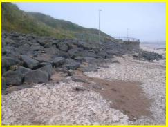
Some flattening of rock revetment at south end of Spittal seawall.
