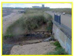
Localised erosion to the dune edge from the outfall constructed in 2009/10.
