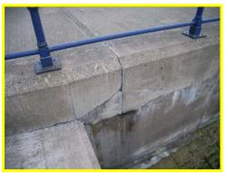
Abrasion and cracking of the South Pier at the junction with Bay View Road.
