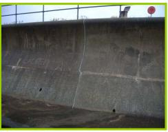
New sealant to joints in recurved seawall.
