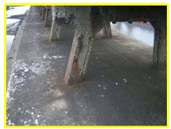
Corrosion and spalling to most of the trestle legs along Blyth East Pier.
