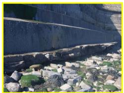
Abrasion, rotting timber wailing and undercutting at toe of seawall.
