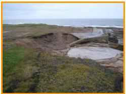
Undermining, outflanking and collapse of south end of low wall.
