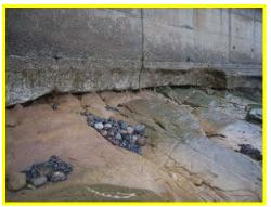
Abrasion of the toe and localised undermining.
