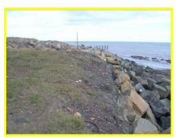
Erosion behind the revetment crest to the south of the Power Station.
