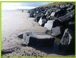
Some displaced rocks along toe of revetment fronting site of old foundry.
