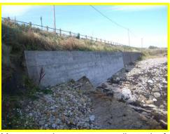
Masonry and concrete seawalls north of Dell Point in fair condition.
