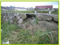
Some localised cracking and missing stones in masonry wall.
