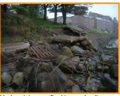
Undermining, outflanking and collapse of Pier Road seawall not worsened.
