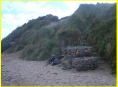
Deformed gabions at access steps and dune blowout north of Beacon Hill.
