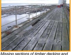
Missing sections of timber decking and rot at some fixings.
