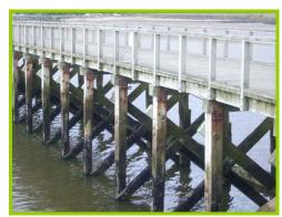
Timber piles and superstructure of South Jetty in good condition.
