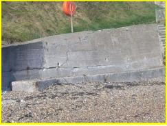
Large horizontal crack along base of concrete section of wall.
