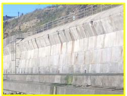
Spalling of concrete along upper section of seawall at north end of Collywell Bay.
