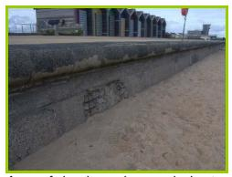
Areas of abrasion and exposed rebar to the seawall at Links Road.
