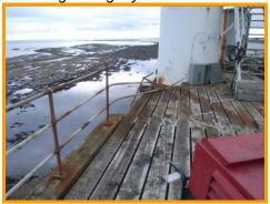
Timber edge beam missing causing collapse of a section of hand railing.
