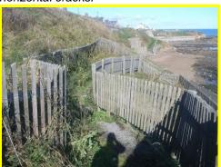
Movement in fencing along the access path above the high seawall.
