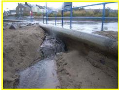
Erosion in the upper beach at the car park access due to run-off.
