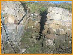
Some small gaps between blocks in wall Void in steps in wall along the inner north bank adjacent to road bridge.
