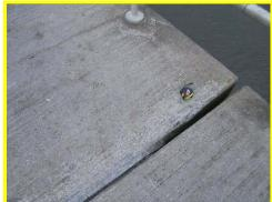
Minor rotation in one deck section in the South Pier Head.
