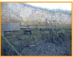
Large gaps and some missing block in lower section of masonry quaywall.
