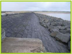
Rock armour and masonry on north face of North Pier in good condition.
