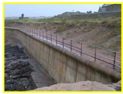
Erosion of the vegetated slope behind Abrasion of the the crest of the seawall at Church Point. undermining.
