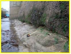
Undercutting of the main wall of Beadnell Breakwater.
