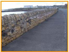
Repairs to crest wall and resurfacing of roadway at Nackers Hole Beadnell.
