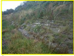
Overgrowth on stone revetment along B1342 overgrown.
