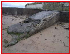
Abrasion, spalling and voids in seawall access ramp.
