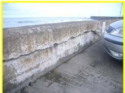
Significant horizontal crack in crest of seawall opposite RNLI building.
