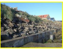
Erosion of earth slopes behind crest and tipping of building rubble.
