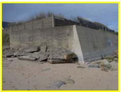
Concrete slurry and rubble along south end of seawall.
