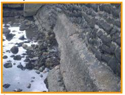
General undermining and potential loss of concrete toe works.
