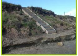
Timber steps moved landward to address erosion in upper slope.
