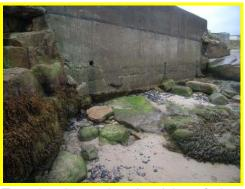
Outflanking and erosion behind the crest Toe abrasion and undermining of short of short seawall north of Newbiggin seawall north of Newbiggin Point.
