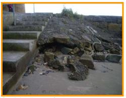
Partial collapse of concrete revetment at north end of Beadnell Bay.
