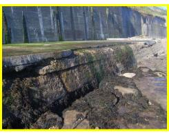
Significant abrasion at the toe and horizontal cracks.
