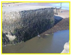
Masonry wall on the west bank of Seaton Burn in good condition.
