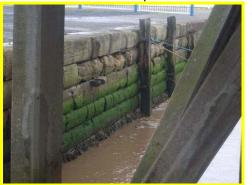
Abrasion and cracking of masonry blocks on east face of Spittal Pier.
