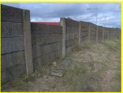
Some broken and missing planks along wall at back of dunes.
